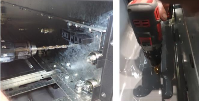
Drill pilot drilled holes to specified diameters
